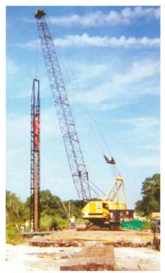
17. The piles will be driven to a factored design load of 630 kN (71 tons) which is about 3 times the estimated required bearing capacity.
